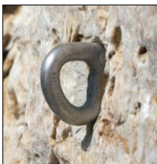
Raumer stainless steel glue-in bolt - good
